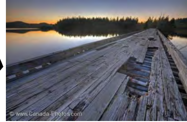
Old Lake Bridge, Vancouver Island
